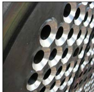
Completed strength weld removal.
