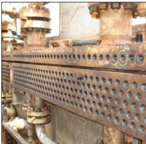
FinFan cooler before maintenance
